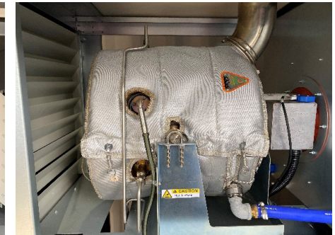
Original vs Modified Capstone C30 Turbogenerator
