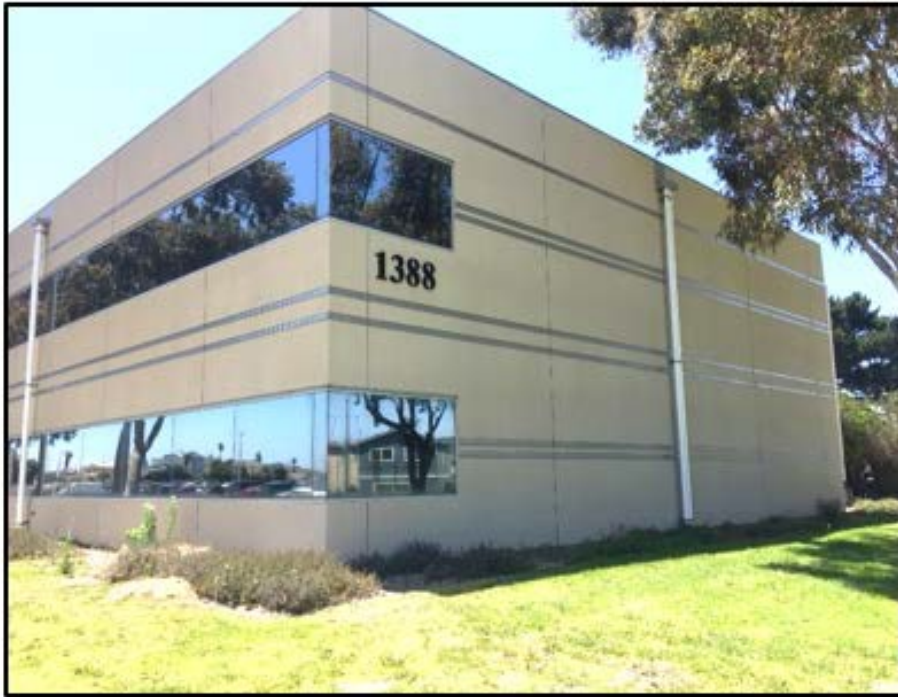
NAVSEA Database Server Farm Building PH1388
